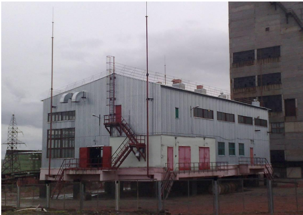
Fig. A.4-5. VPS-3 is the first completed facility within the framework of the methane utilization project at Severnaya Coal Mine of OJSC "Vorkutaugol"
