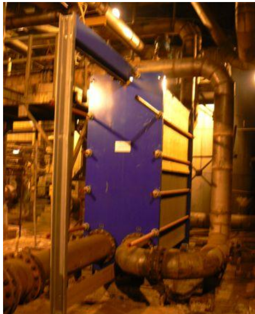
Fig. A.4-4. Plate heat exchanger erected in the Bleaching-and-Cleaning Department
